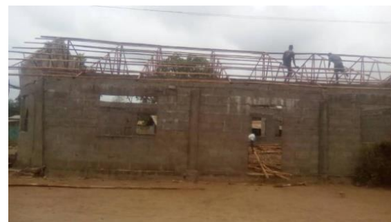
Roofing Work in progress at Baptist Church, Lungi
